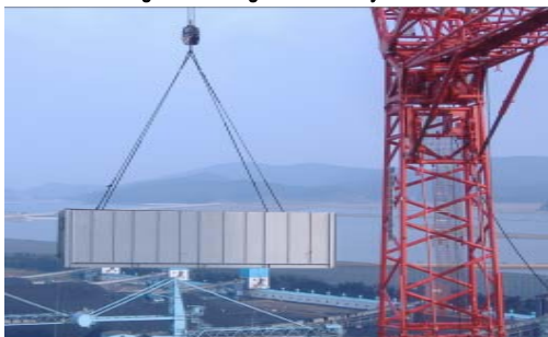
4.3 Lifting Second Site Ass'y
