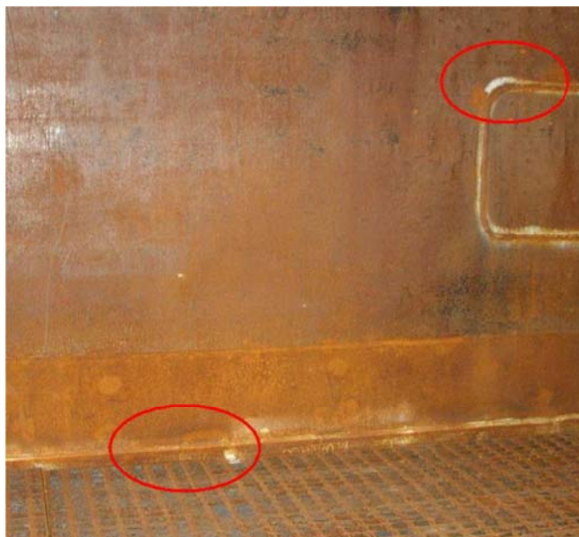
Fig.4 Problematic floor/wall junction an welding on wall
