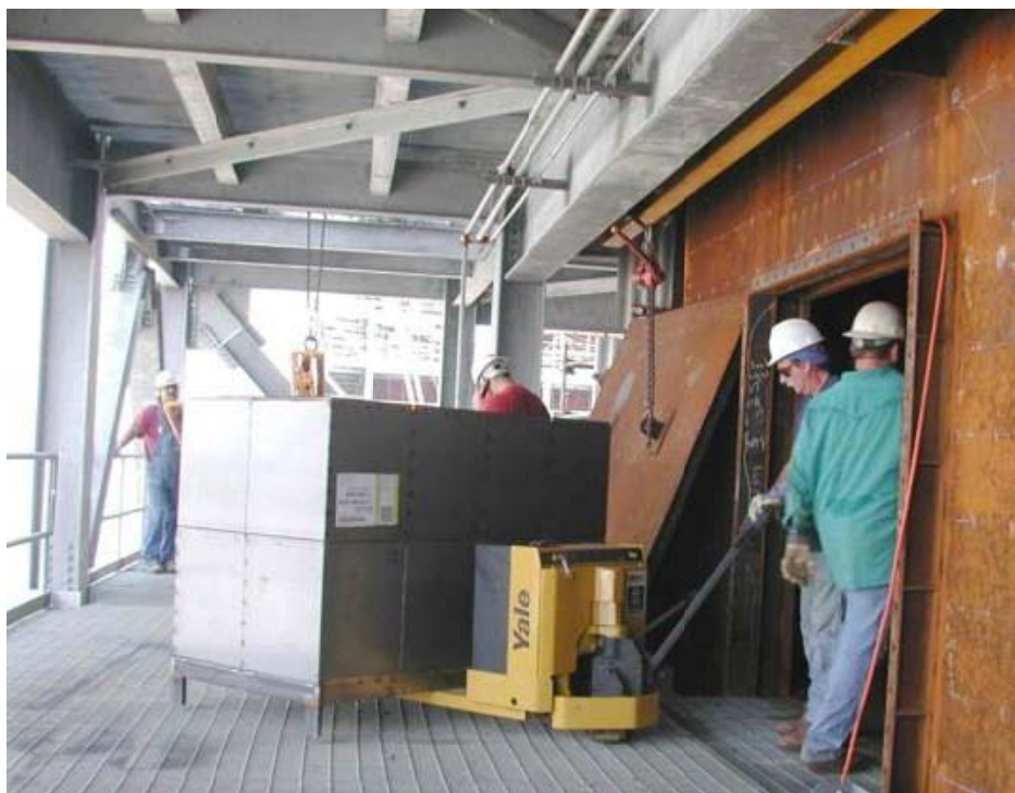
Fig. 12 Transport of modules into the reactor using a pallet car.
