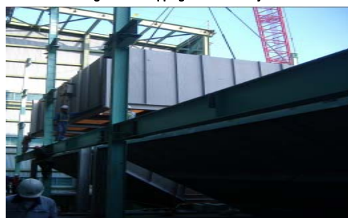
Figure 4.4 Dropping Second on First Site Ass'y.
