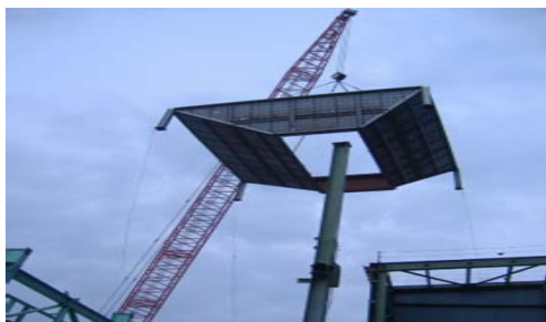
Figure 4.1 Lifting First Site Ass'y
