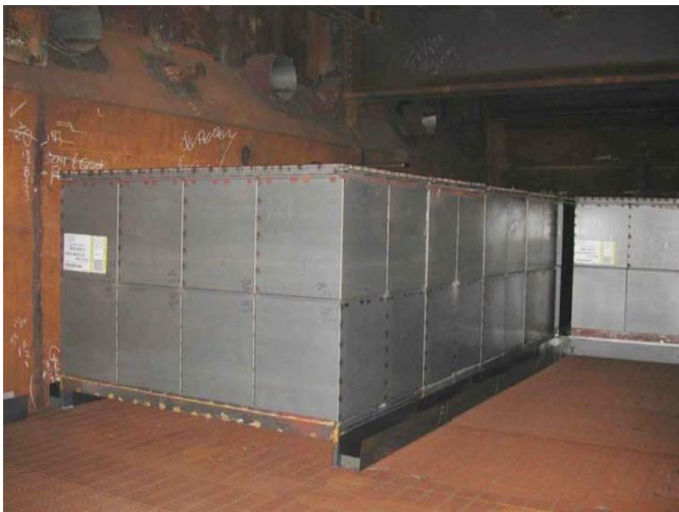
Fig. 13 Sealing gutters between modules
