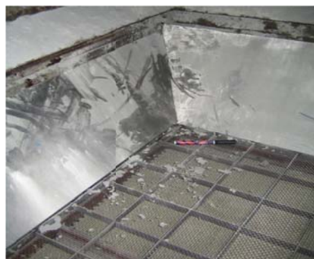
Fig. 9 Dust deflector in corner, cut to fit.
