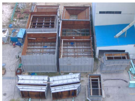
Figure 3 Site Assembly of SCR duct and reactor
