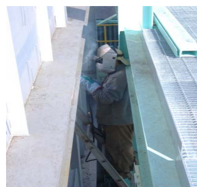
Figure 5.3 External Connecting between site ass'y parts
