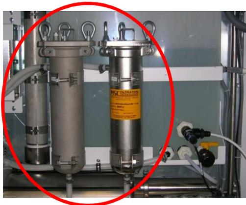
**Figure 24 - Guard Bed Housing Assemblies Location**
