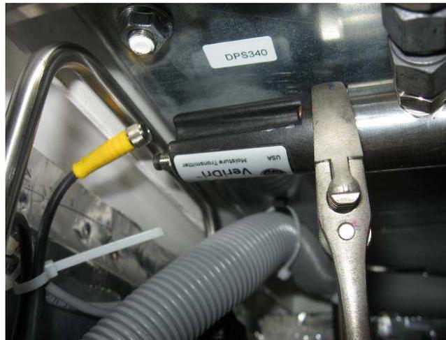
**Figure 53 - Dew point sensor replacement**
