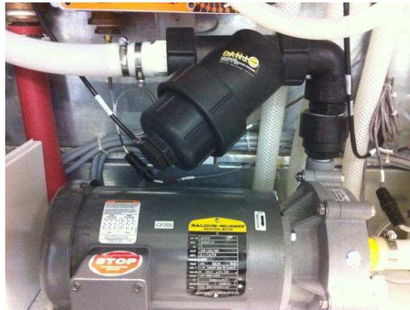
**Figure 21 - Strainer Housing Locations**
